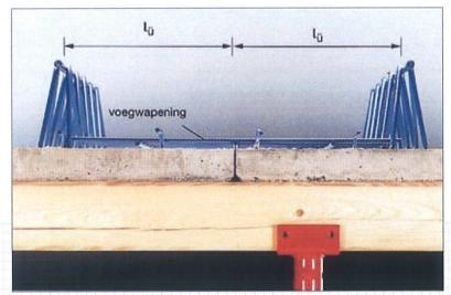
The distribution of the extra reinforcement is shown on the construction diagram. Such additional reinforcement is normally provided for exchanges, transversely placed slabs and the like. The top reinforcement of the base slab is described in a separate reinforcement plan. This is required as top reinforcement for contiguous fields, overhangs, etc.
